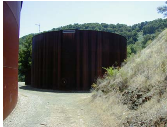
NEARY NO. 1 TANK EXTERIOR
